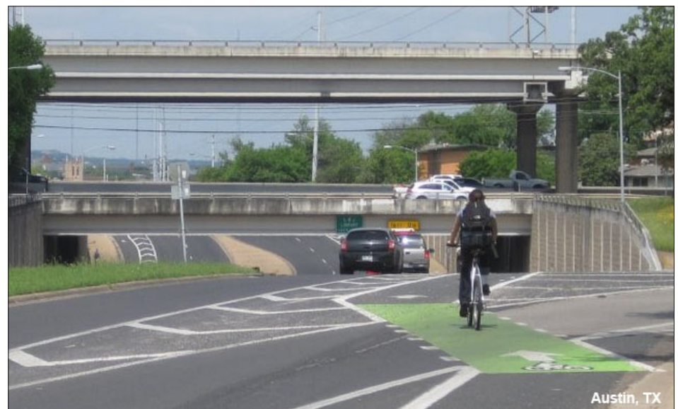
Bike lane treatment at a freeway on-ramp in Austin, TX. (Photo: Courtesy of NACTO)
