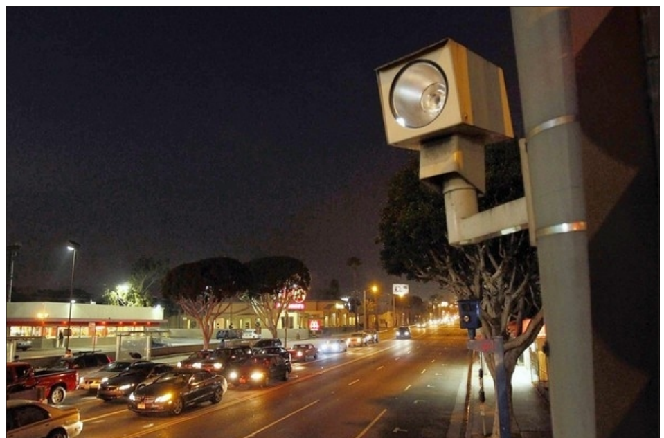
A red light camera installation. (Photo: Courtesy of TTI)
