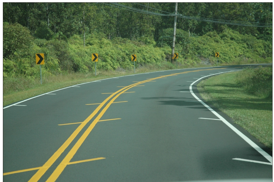
Sharks' teeth installed along a high-accident location on Big Island, Hawaii. (Photo: Courtesy of Aaron Takaba, Hawaii County Department of Public Works)
