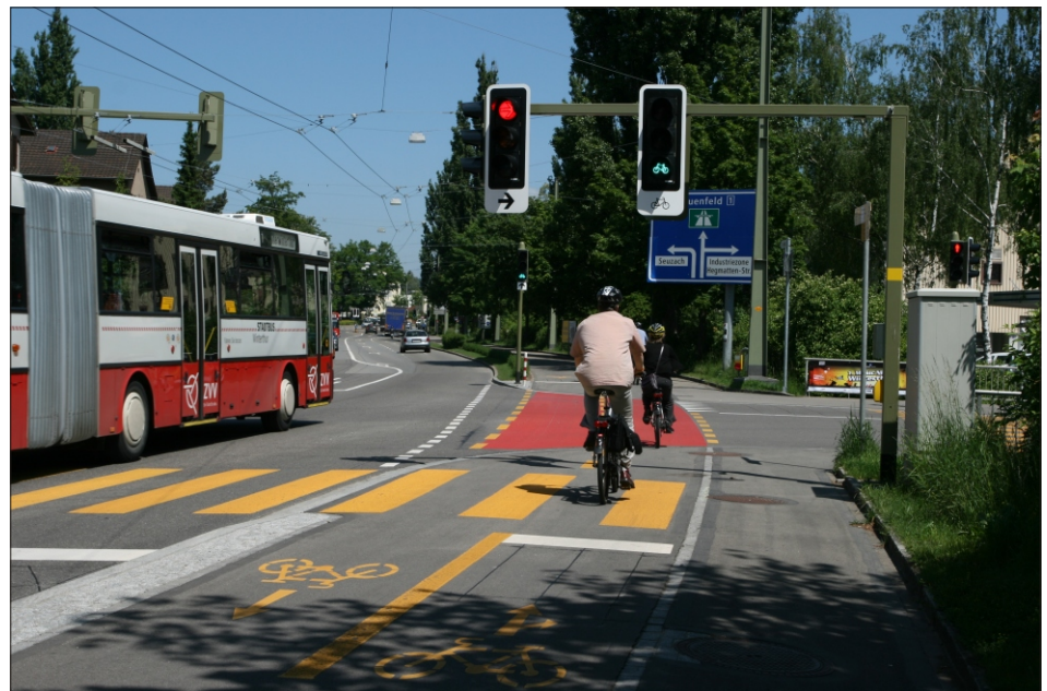
A separated bikeway in Winterthur, Switzerland has bicycle signals and painted pavement to reduce turning vehicle conflicts and improve intersection safety. (Source: FHWA International Scan report)
